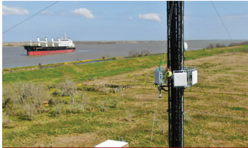
Louisiana - 5G antenna install
